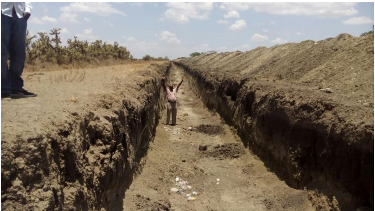
Plate 3: Showing the depth of the moat in segera ranch
