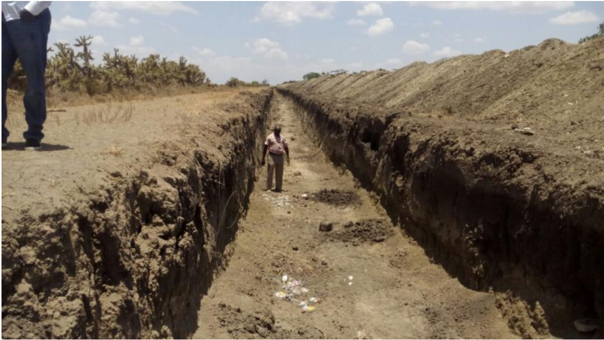
Plate 2: A section of the moat in segera ranch
