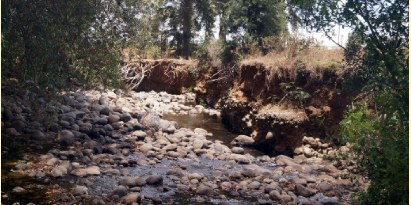
Nanyuki River: effects of degradation
